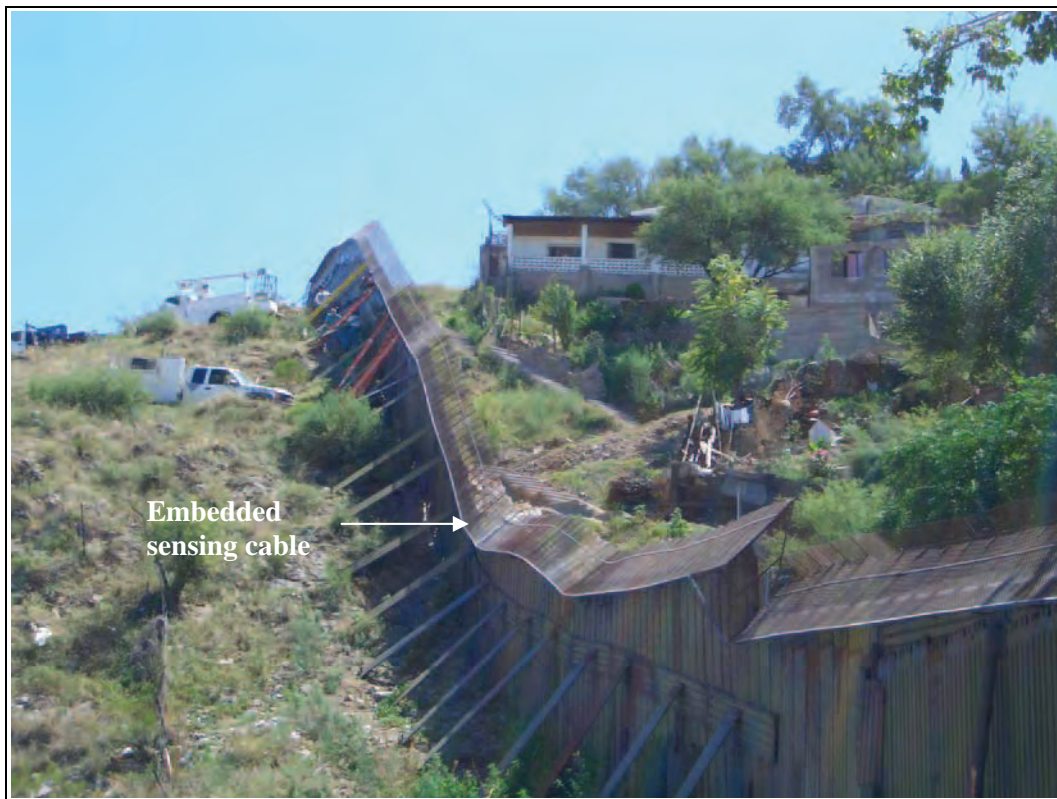
Fig. 7 FFT Secure Fence system on US–Mexico border. The fiber sensor is embedded within a conduit.
